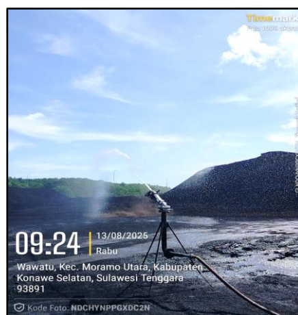
Figure 2. Water spray system in coal stockpile area
