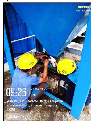
Figure 6. Routine cleaning of dedusting system
